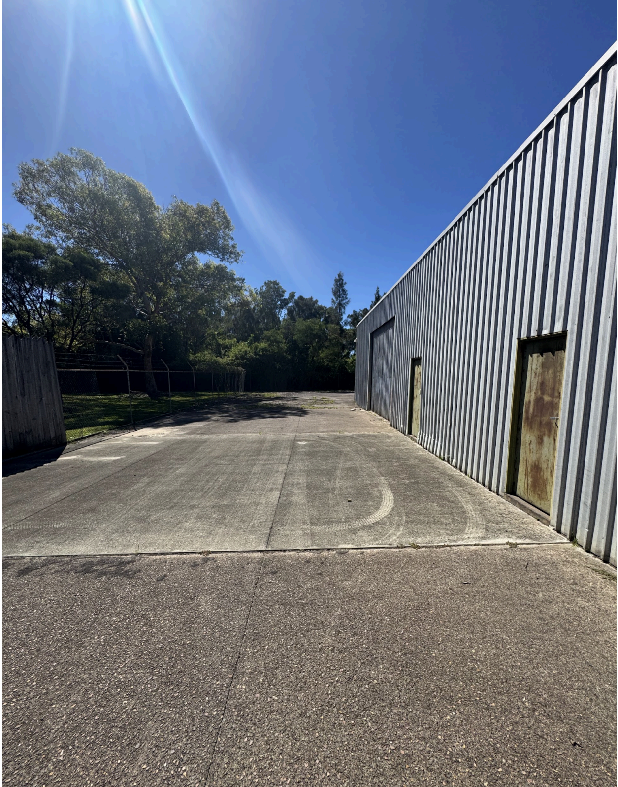
Plate 2: Photograph demonstrating the limited vegetation present on site as well as one of the two industrial sheds proposed for demolition.
