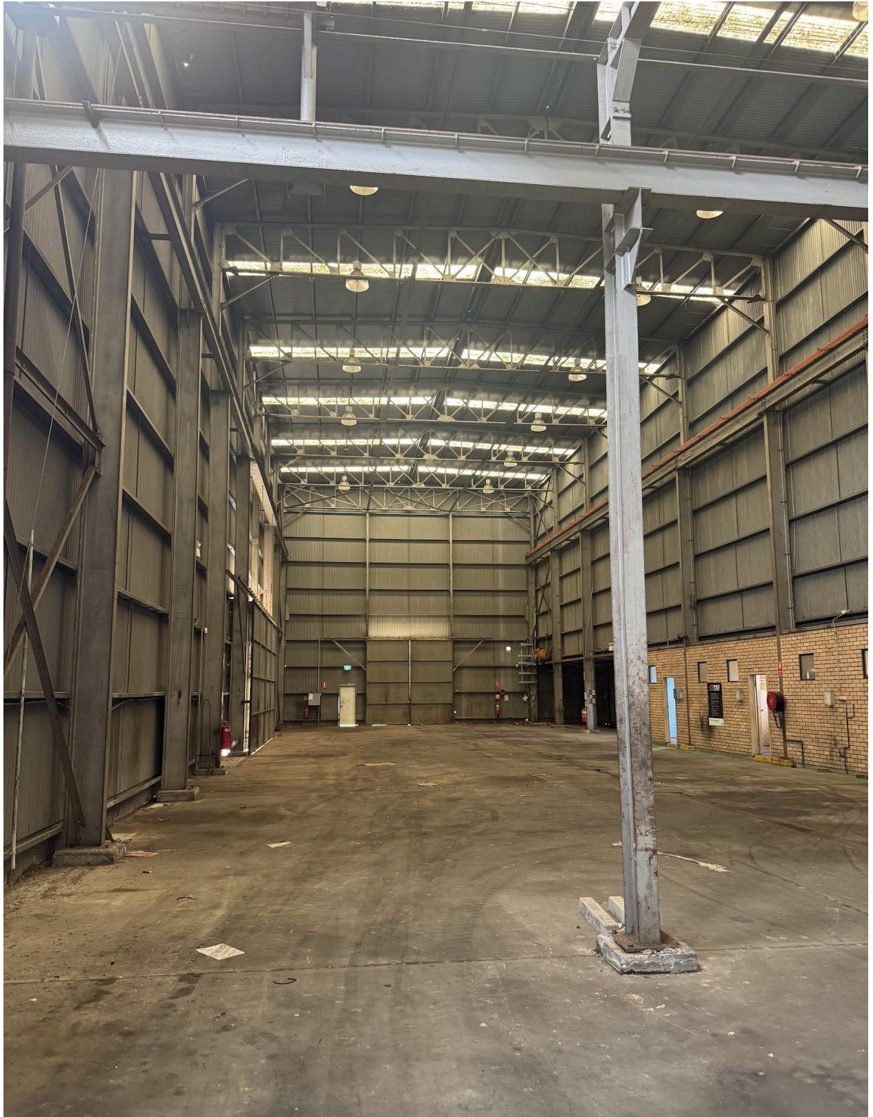
Plate 4. Internal survey of the southern shed
