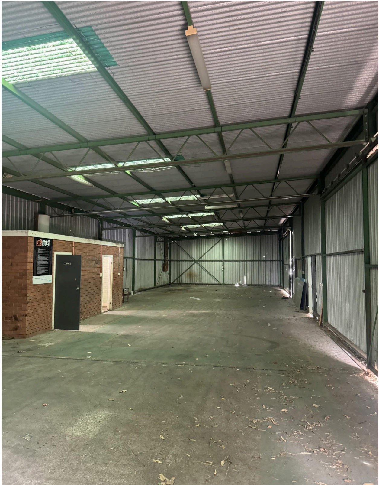
Plate 3. Internal survey of the northern shed.
